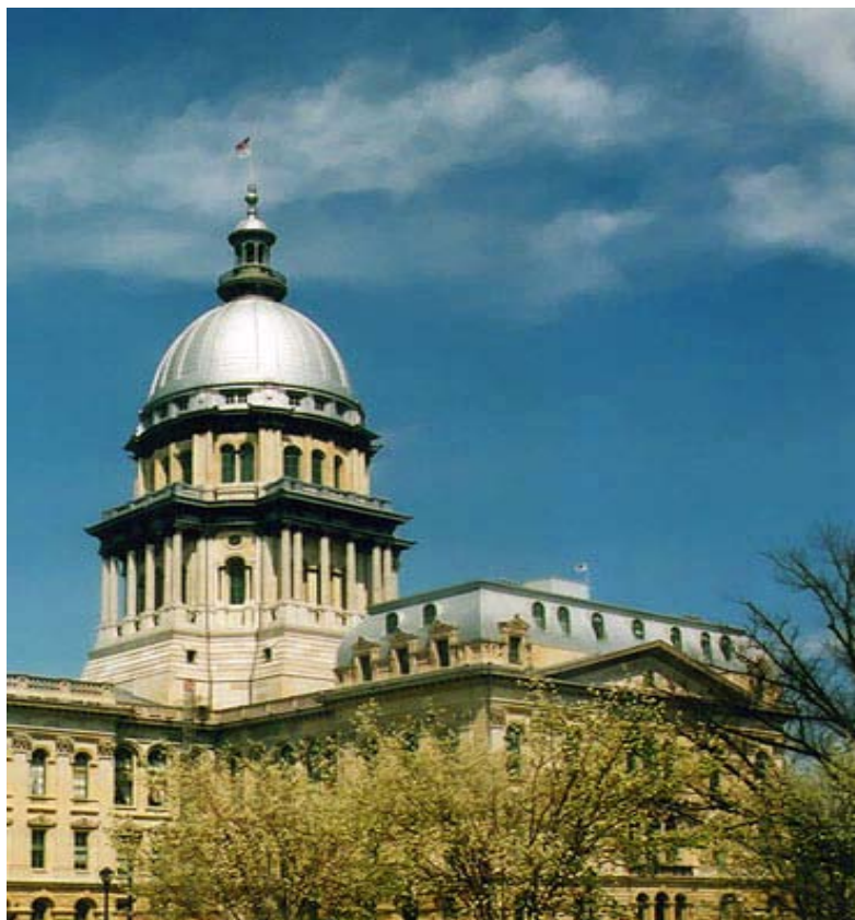
Illinois State Capitol Building
